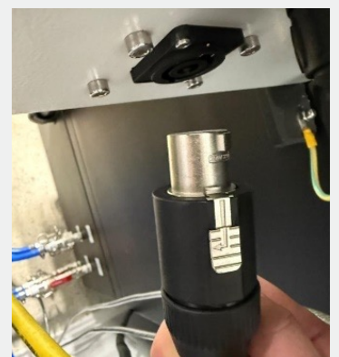
Figure 6 Single-phase Electrical Connection
